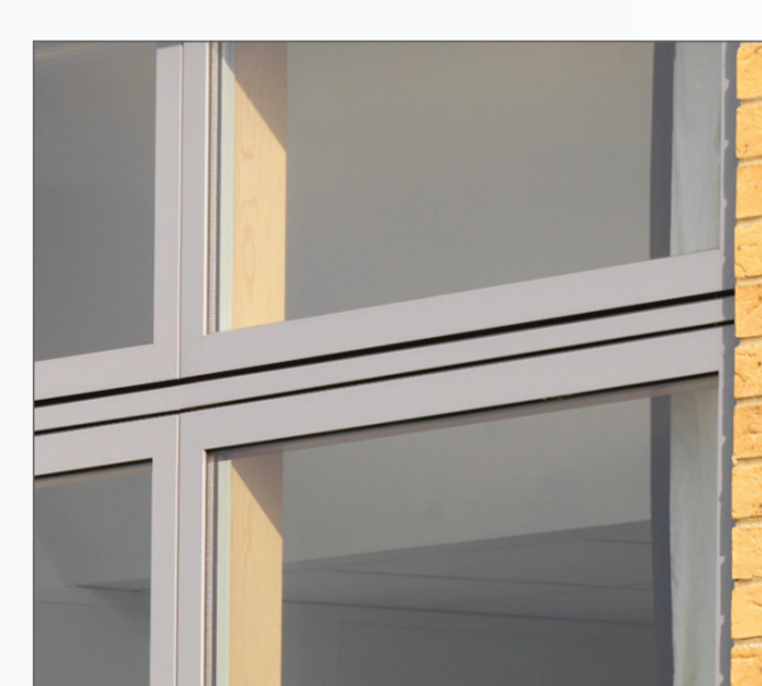
Ventilation position. The striking plate allows a 5mm night ventilation opening for all espagnolette handles.
